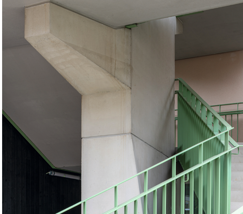
Enjoy Concrete's precast elements feature sharp edges in exposed concrete quality.
