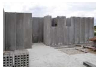
Erected partition wall panels
