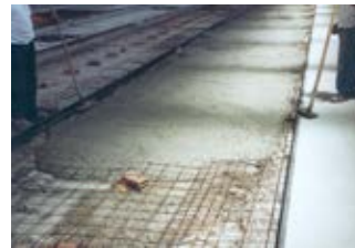
Concrete bed preparation
