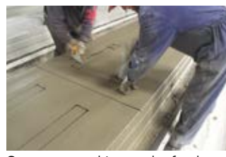
Operators working on the fresh concrete marked out by the plotter
