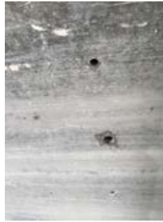
Detail of weep holes at the bottom surface of the concrete element
