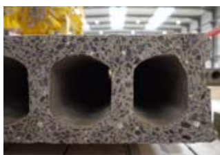
Excellent concrete compaction and steel wire bonding
