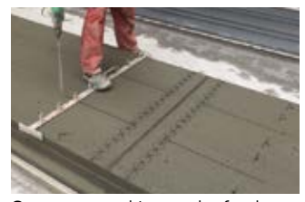
Operators working on the fresh concrete marked out by the plotter
