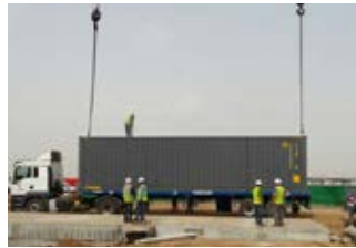
Installation of the heating plant container
