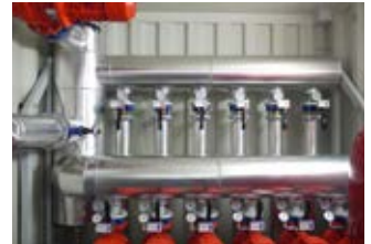
Primary pumping circuit manifold
