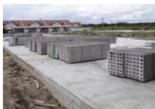
Partition wall panels on-site
